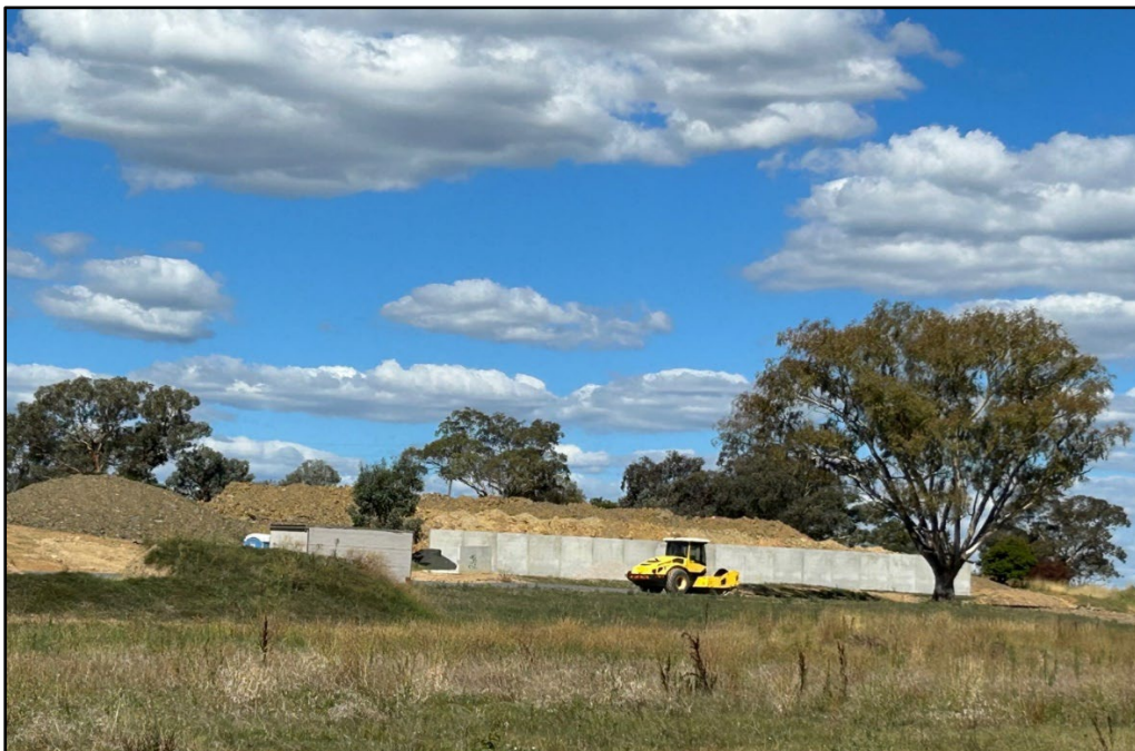
Photo 2: Subject site (further west from Photo1) looking toward the northern boundary showing current earthworks being undertaken and approved under DA0233/2022
