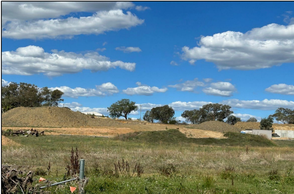
Photo 1: Subject site looking toward the northern boundary showing current earthworks being undertaken and approved under DA0233/2022
