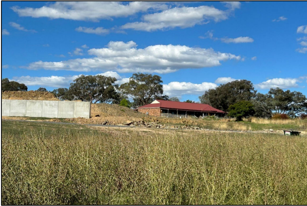
Photo 3: Subject site (further west from Photo 1 and 2) showing extent of current earthworks and the existing dwelling to be used as a managers residence
